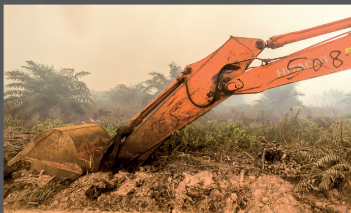
Excavator on plantation in Central Kalimantan, Indonesia, September 2015 © Victor Barro/FoE
